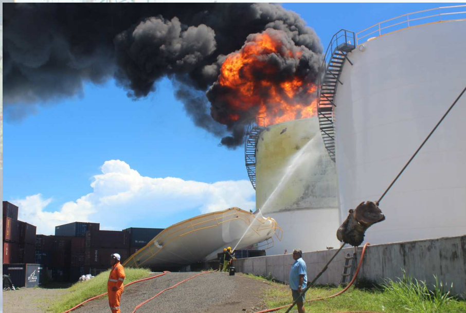
Samoa, 4 april 2016, dieseltank (Ø 15 meter)
