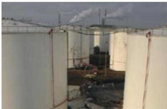
Fig 7.2 – Loss of containment, fixed roof tank
