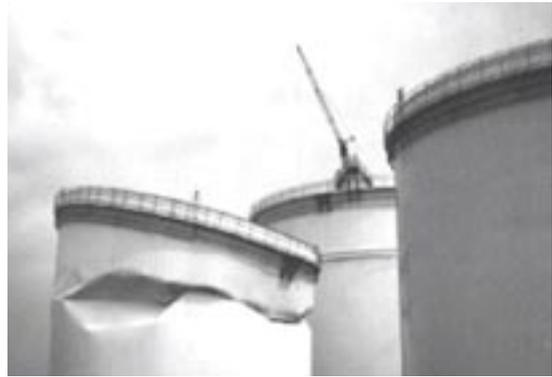
Fig 5.7 – Example of a tank collapse due to internal corrosion which was not detected properly.
