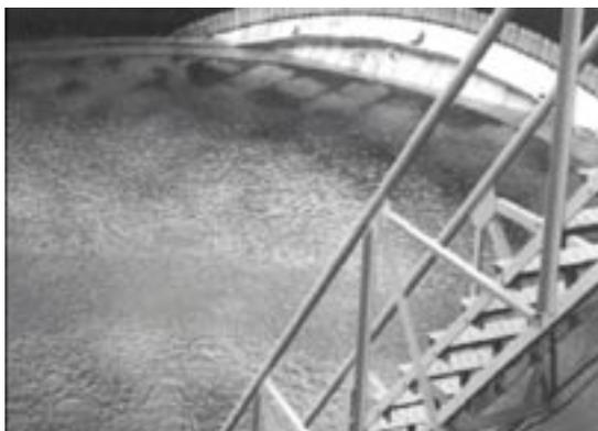
Fig 5.6 – Example of a sunken floating roof – caused by roof overloading
