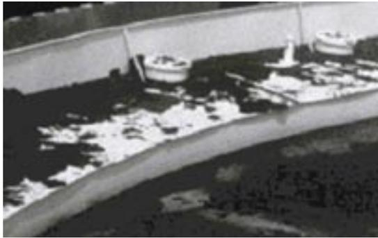
Fig 5.4 – Corrosion, waxy crude deposits and waste on a floating roof will lead to blocked roof drain, which in turn will load the roof and lead to roof sinking.
